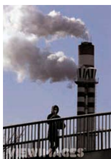
..... are coming out of the chimney.
